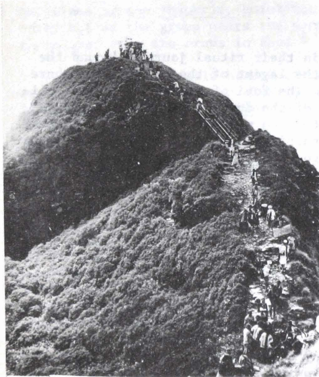
6. The stair-bridge to the top.
